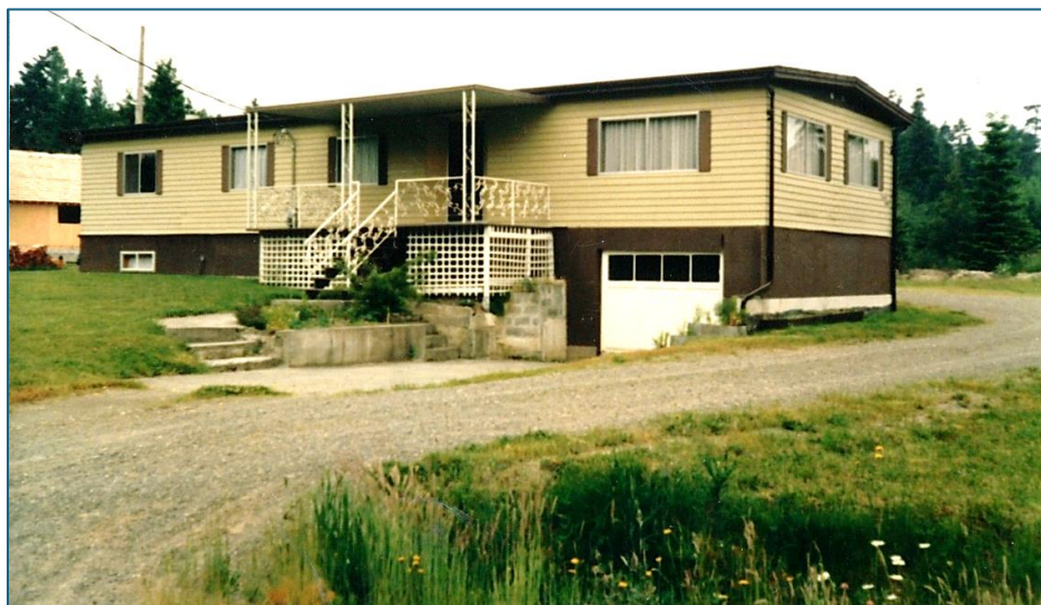
The double-wide trailer, 1978. Today it is a private residence (775 Wembley Road).
